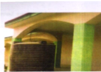
Plate 4: RHW Collection Tech. Source: Field Survey 2018
