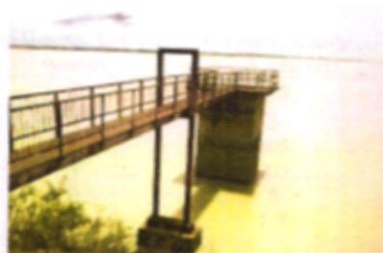
Plate 7: Gari Dam Reservoir Source: Field Survey 2018
