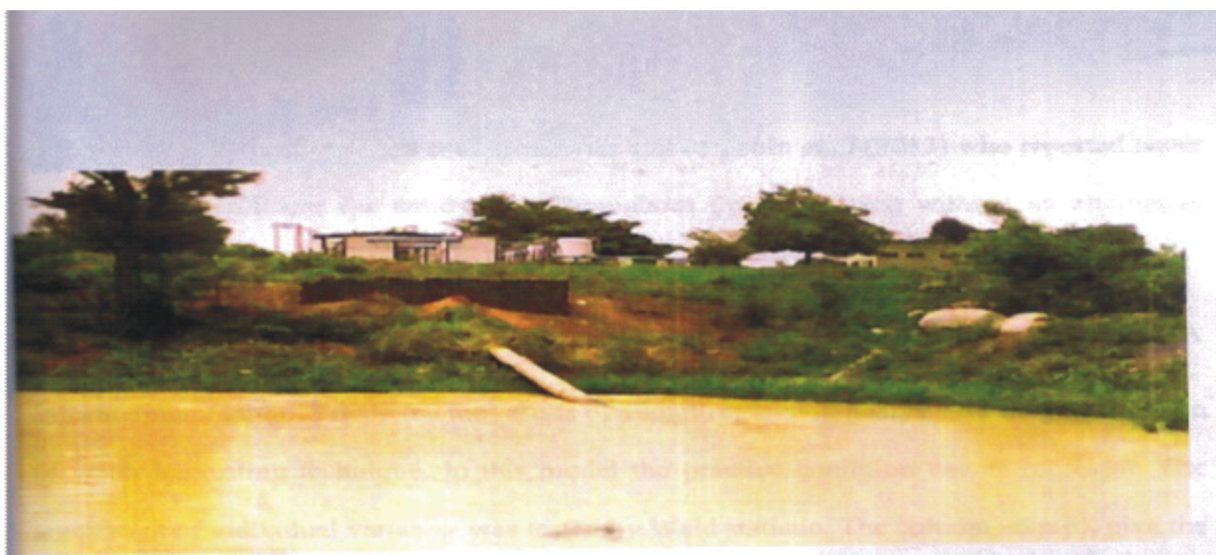
Plate 12: Treatment site preparing & supplying water from Gari Dam for households uses Source: Field Survey 2018
